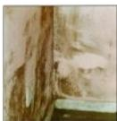
Condensation mould photo for illustration purposes only Mould growth will appear on any damp surfaces such as plaster, wall-paper and timber and is associated with condensation problems in many buildings. It is unacceptable because of appearance (unsightly growths of various colours greens, yellows, pinks, black, grey or white)
